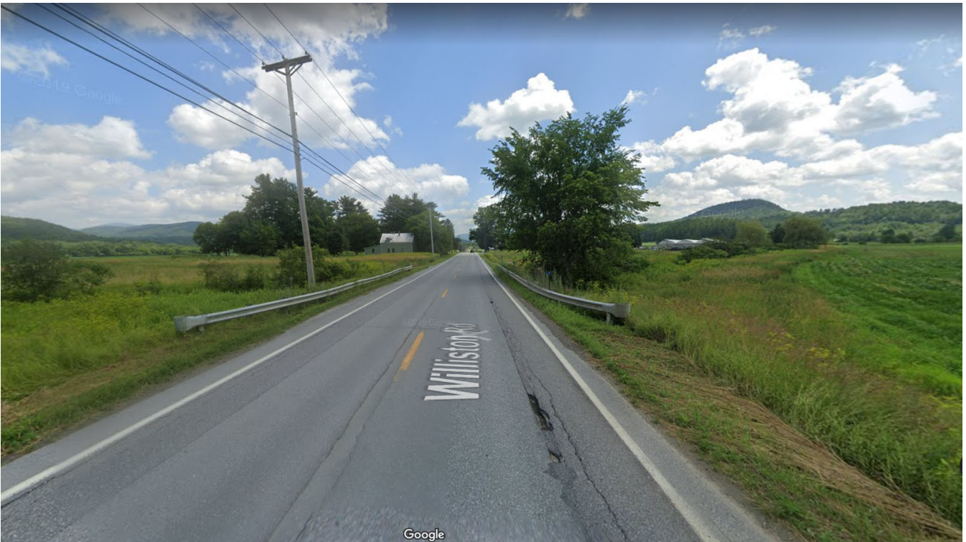
Looking East over Culvert 23
