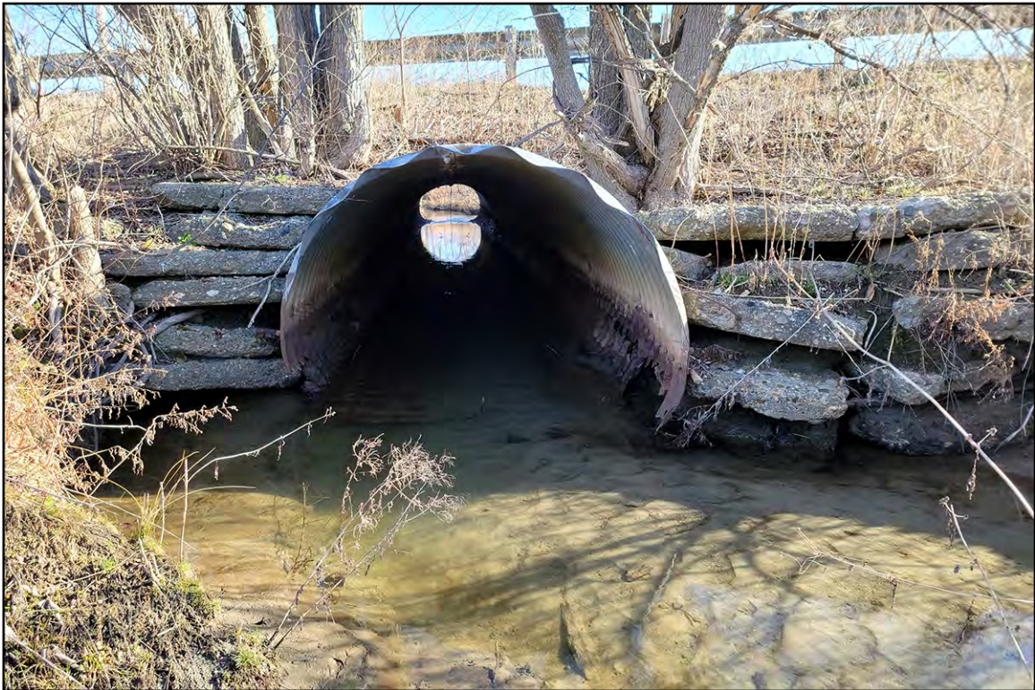
PLATE 3: Built-up Wingwalls of West Side of Bridge, View East
