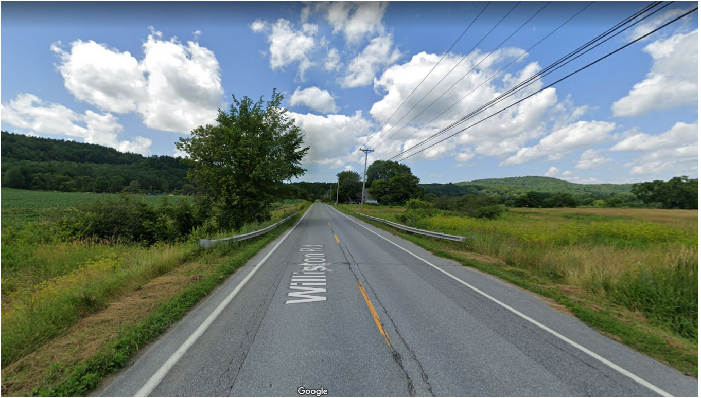
Looking west over Culvert 23
